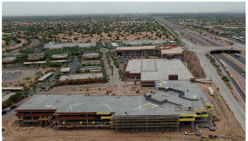
Aerial (facing south) of RCA under construction
